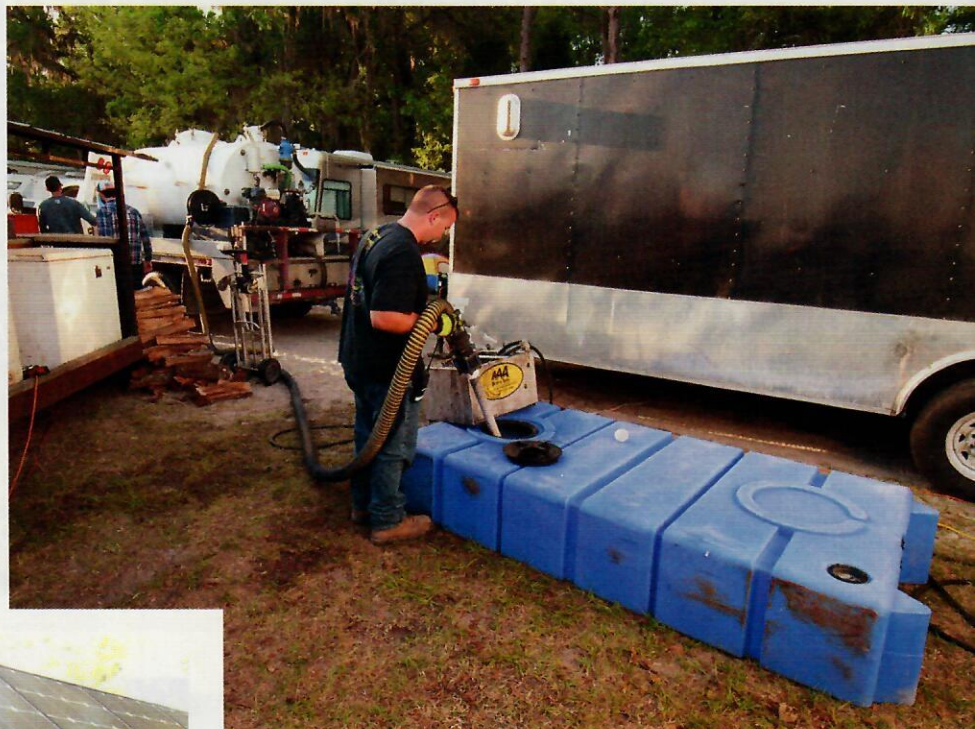
Above: Technician Dustin Fletcher pumps a Kentucky Tank holding tank at the festival. A strainer box built by AAA Porta Serve is seen on top of the tank. It is used to keep rags and kitchen debris out of the holding tank.
